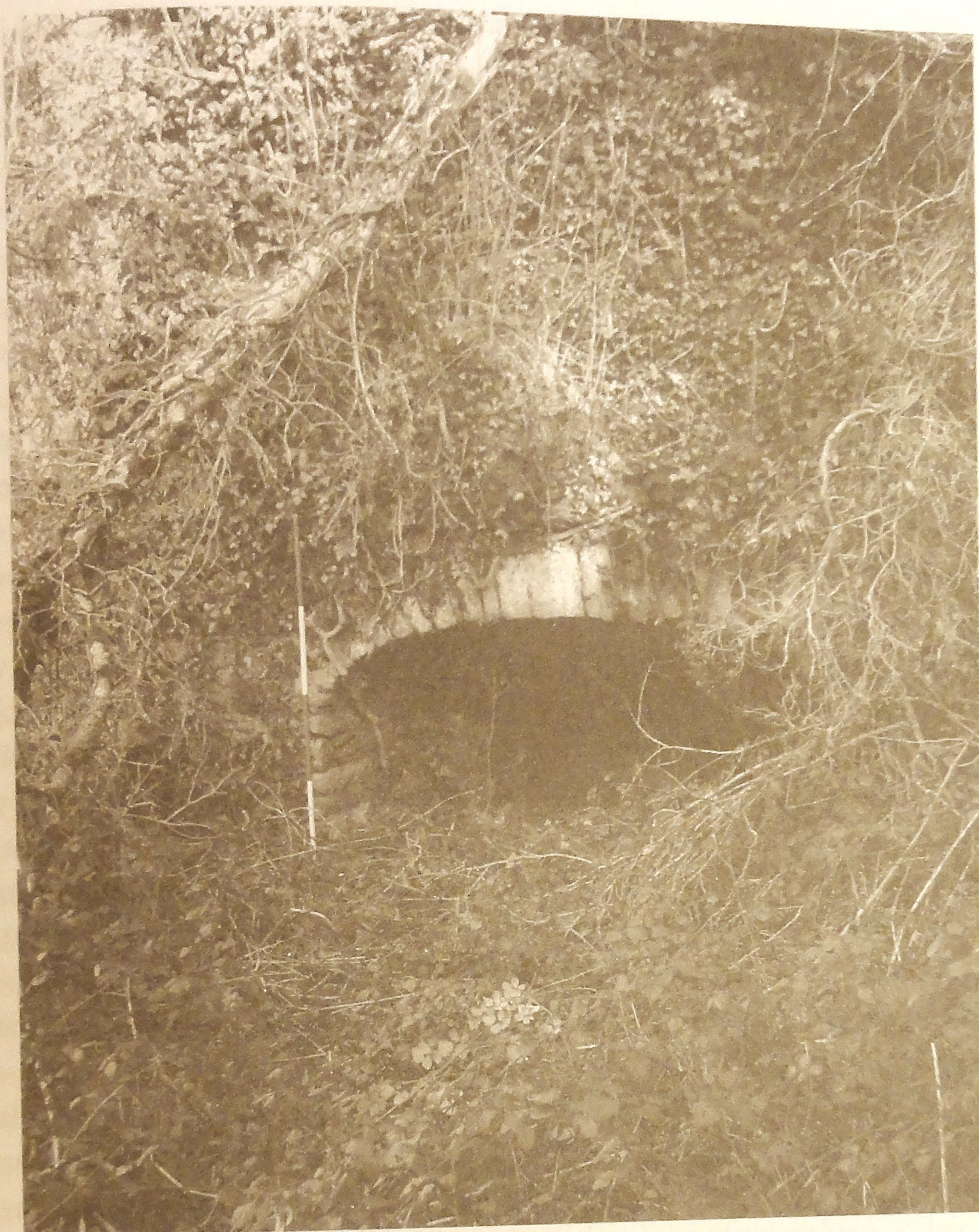
6.2 Standing remains of furnace of c. 1623 at Araglin, Co. Cork (photo: Colin Rynne).
