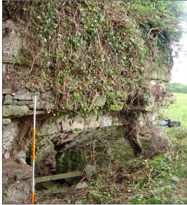
Fig. 8. Blowing arch in the south wall
