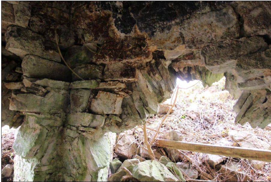
Fig. 18. Internal damage to South arch
