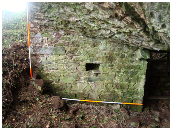
Fig. 6. Recess in the southern tapping arch wall
