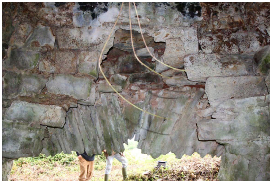
Fig. 15. Damaged interior of the East arch
