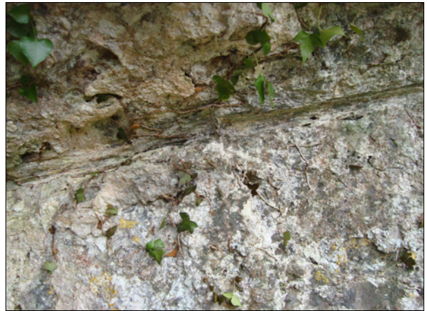
Fig. 8. Imprints of timber/wattle in the western tapping arch wall
