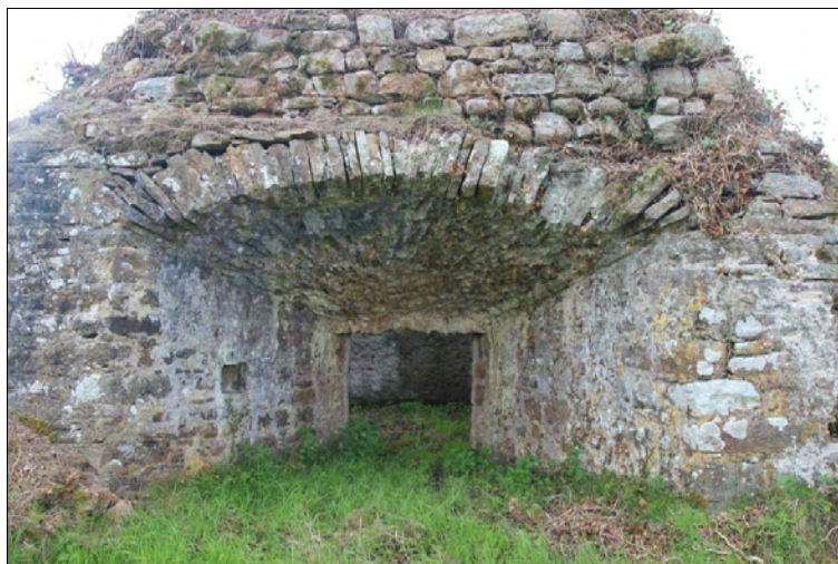
Fig. 13. North wall showing damage to the arch
