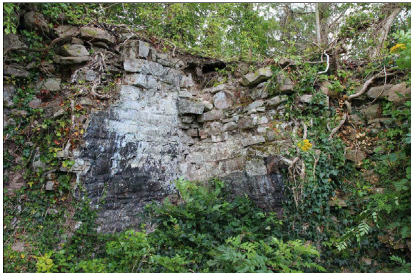
Fig. 25. Exposed inner lining of the furnace
